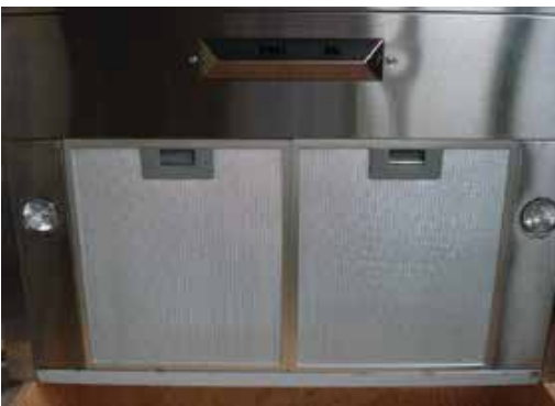
4. Install the mesh filters
